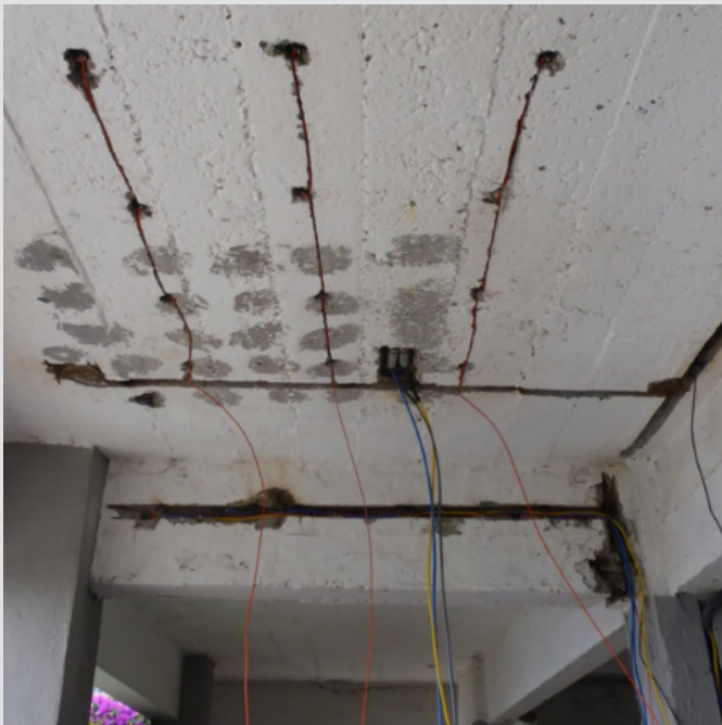
Fig. 3 and 4. ICCP installation and final appearance
