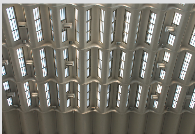
Fig. 2: Particular of the prefabricated elements of the half dome, Hall B (F. Pasqual, 28/01/2020)
