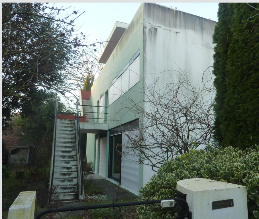
Figure 2: Cité Frugès, free-standing housing called « Maison Vrinat », 4 rue des Arcades, Pessac. Cracks and biological coverings are present on the facades. 2022 © FLC/ADAGP
